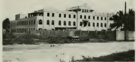
Presbyterian Hospital, San Juan, Porto Rico; the new building now nearing completion.
